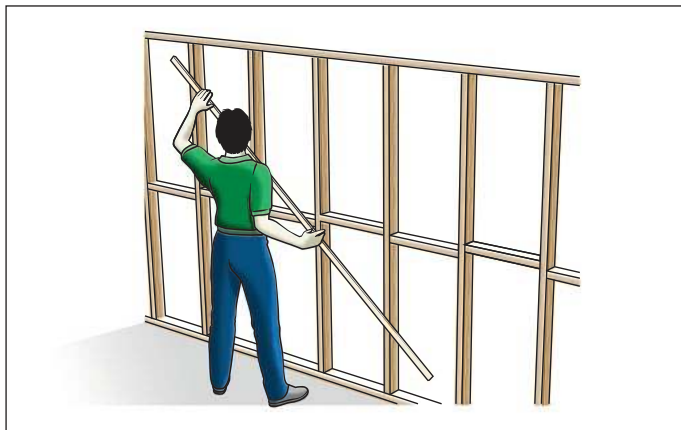
FIGURE 1 FRAME STRAIGHTNESS
