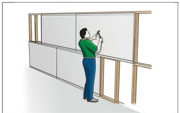
FIGURE 5 FIXING REMAINING SHEETS
